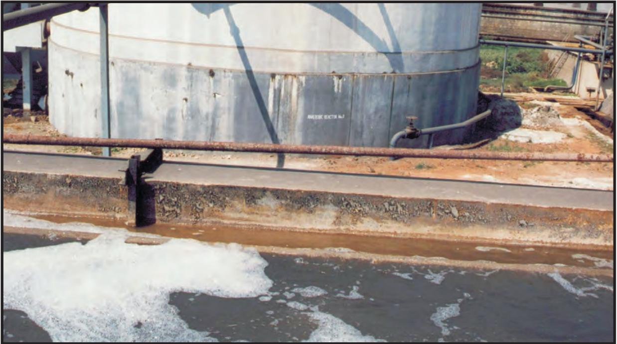
New anaerobic counter current digester 70 M<sup>3</sup>/hr. and preareation tank outlet
