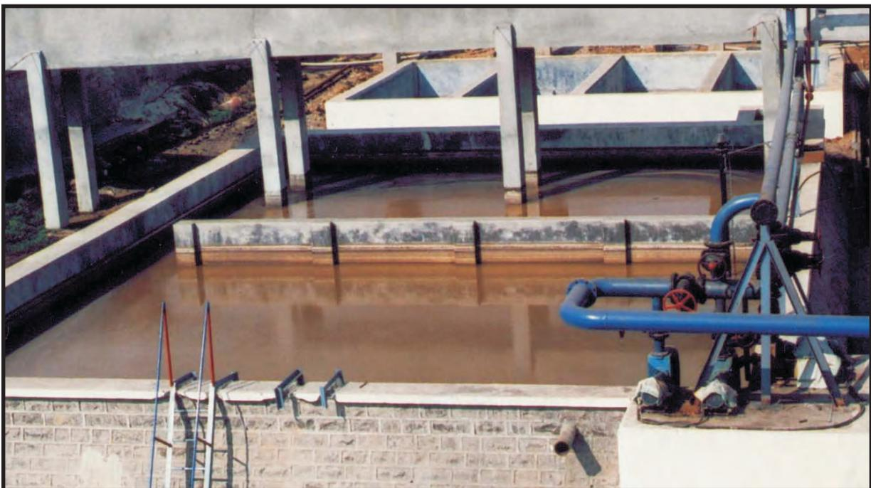
New equalization tank and feeding system to old and new stream
