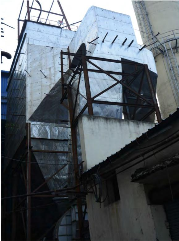
Electro Static Precipitator for
