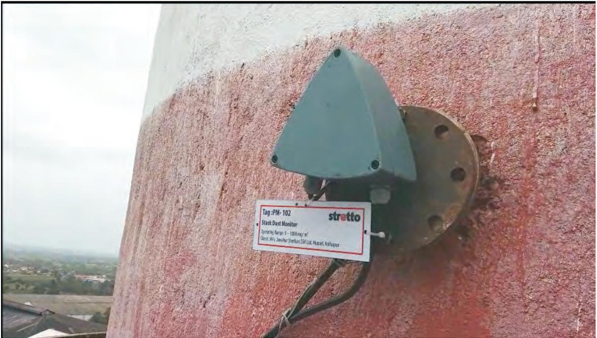
Dust monitor unit for Total Particulate Matter for stack
