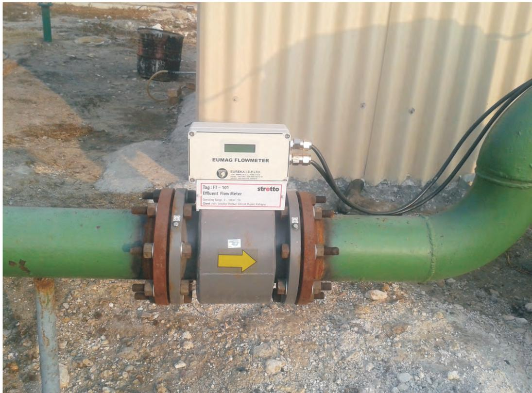
Flow meter for outlet Treated Water
